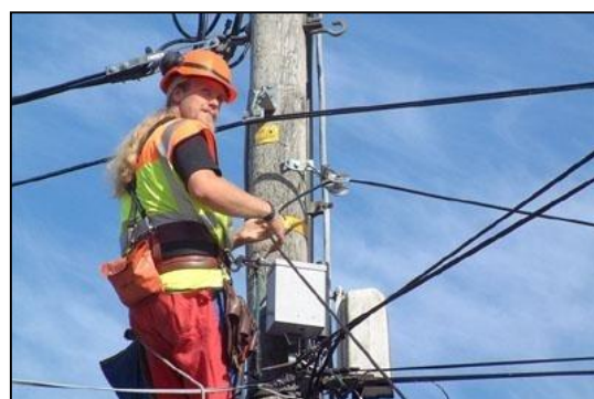
Figure 100: Aerial cable installation
