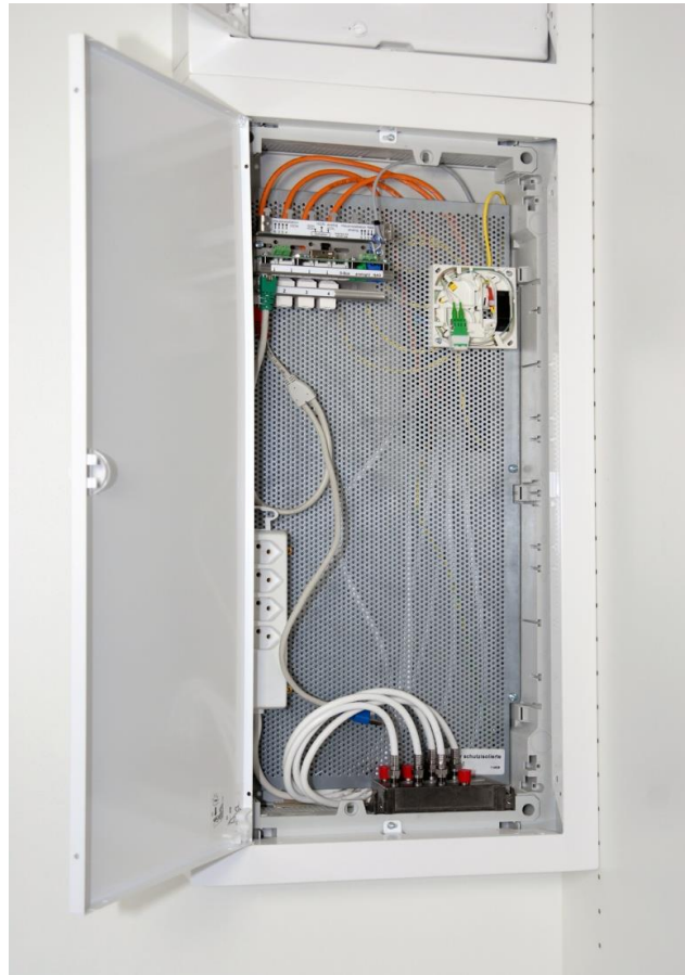
Figure 60: OTO integrated in a home distribution cabinet
