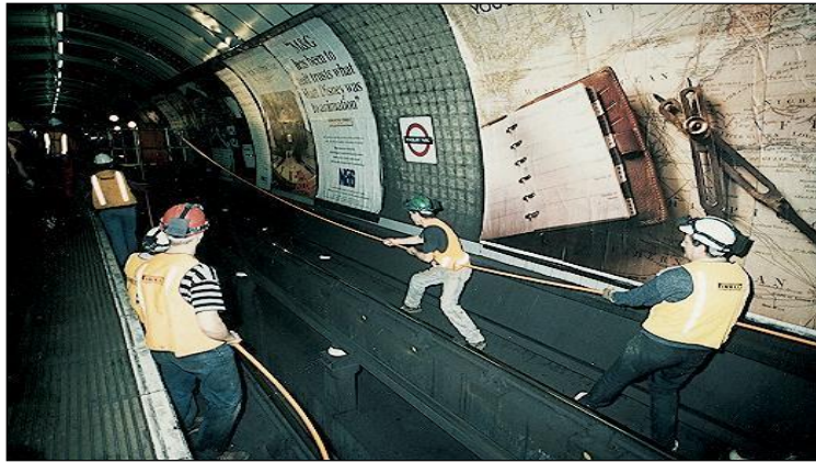
Figure 108: Cable installation in a train tunnel
