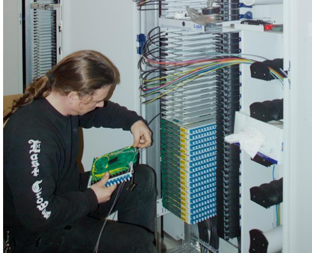
Figure 111: Splicing work on an ODF
