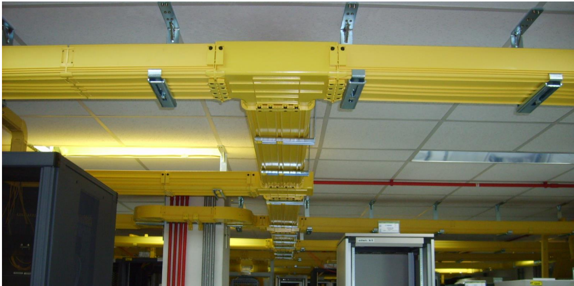
Figure 115: Examples of overhead fibre containment
