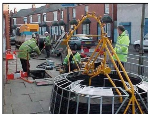
Figure 70: Deploying duct infrastructure
