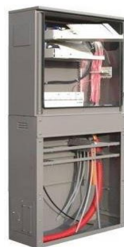
Figure 104: Fibre management
