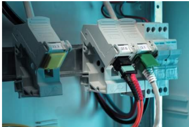
Figure 61: OTO integrated in the home electrical distribution panel
