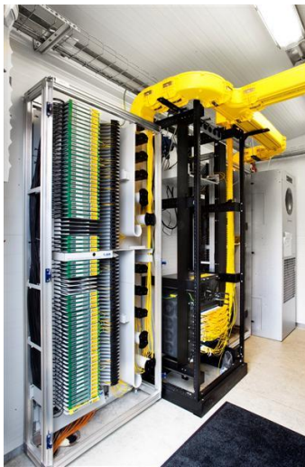
Figure 112: Active and Passive ODF's in a POP
