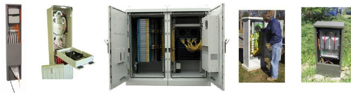
Figure 105: Examples of street cabinets in a range of sizes
