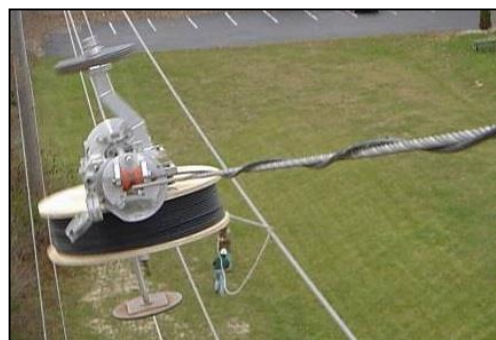
Figure 98: Wrapped aerial cable
