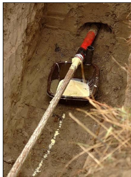
Figure 79: Cable de-coring
