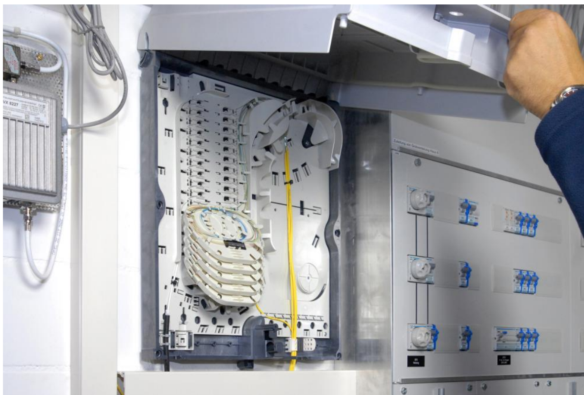
Figure 56: Example of wall mounted BEP installed next to a power distribution
